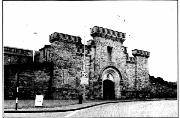
Wexford County Hall, set for refurbishment.
